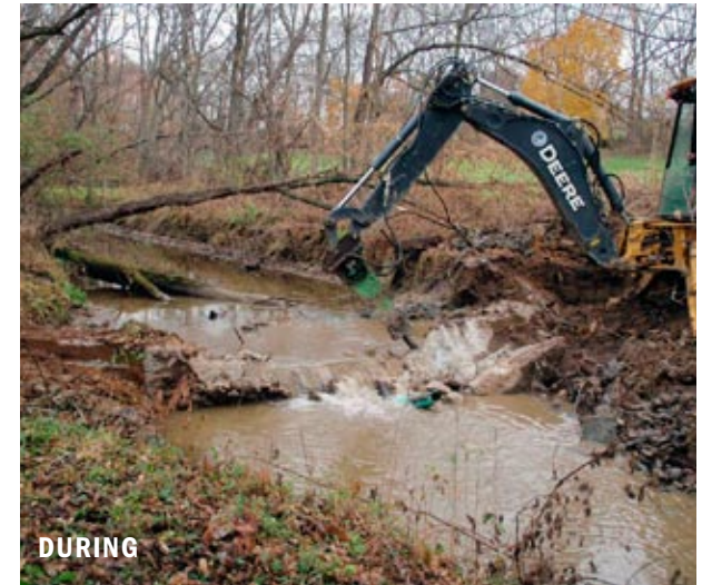
Construction crews carefully remove the dam on the West Branch of Little Conestoga Creek.
