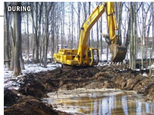
Once the Charlotte Dam was removed, the county recreated the natural meander of the stream. It also installed 30 in-stream structures to create grade control and improve fisheries habitat.
