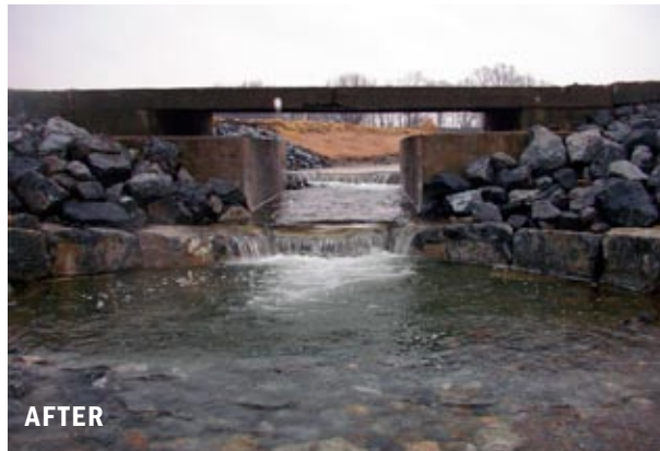
After the removal of the concrete and masonry dam, the stream banks were stabilized, creating plunge pools and making fish passage feasible along the West Branch of Little Conestoga Creek.
