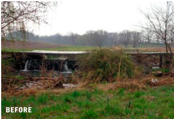
Dam 2 was a concrete and masonry dam located on the West Branch of Little Conestoga Creek. The dam was located under a bridge crossing.
