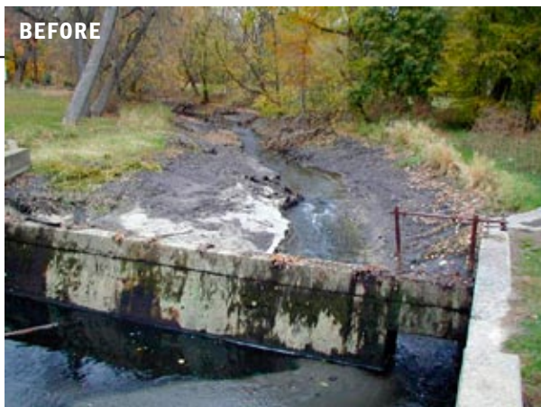
The Charlotte Dam was built to provide cooling water for a steam-generated water works facility. To remove the dam, the county sectioned it into four pieces.
