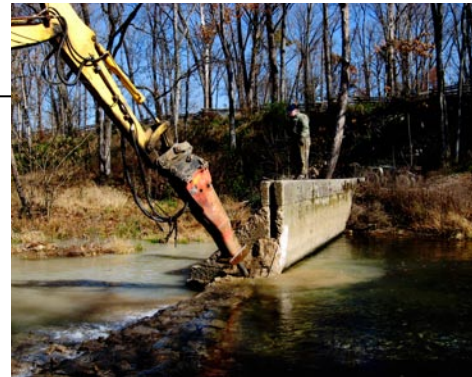
Restoration partners use heavy equipment to remove the Sandy Hook Dam.
